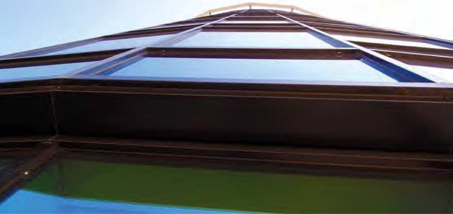
Blue Towers, Ghent
